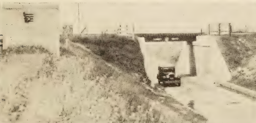
FIGURE 1.—TYPICAL UNDERPASSES REQUIRING DRAINAGE BY PUMPING. NOTE WATER STANDING IN ROADWAY IN THREE OF THE PICTURES.
